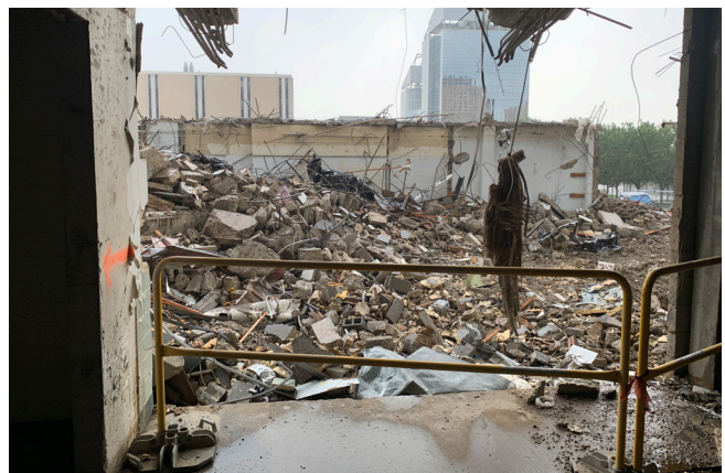
Renovation of Crouse Hall
