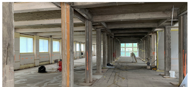
Third floor of Crouse Hall during reconstruction
