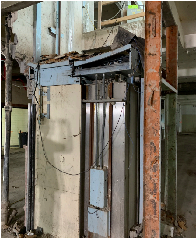
Photo of elevator during Crouse reconstruction
