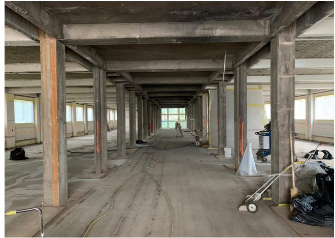
Fourth floor of Crouse Hall being renovated
